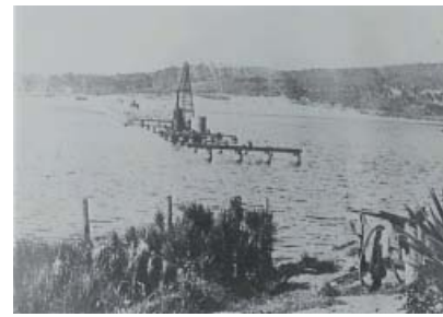
1925 - Ocean Street Bridge Construction
